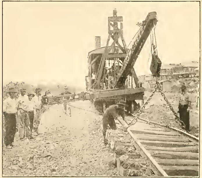
THE TRACK SHIFTER IN ACTION
